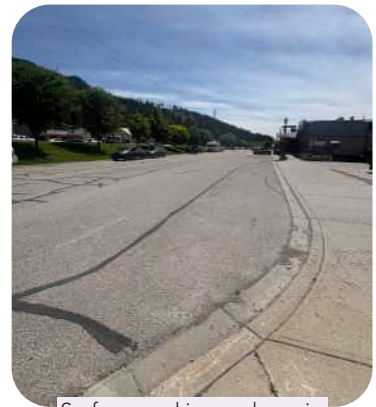
Surface cracking and repair
